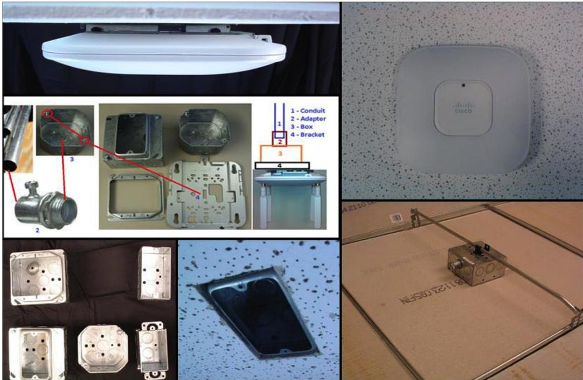
Mounting an AP onto an electrical conduit box (ceiling T-bar or conduit)
