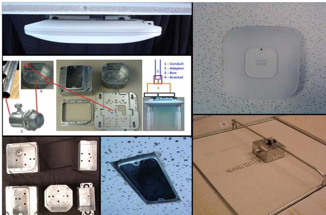
Figure 65. Mounting an AP onto an electrical conduit box (ceiling T-bar or conduit)
